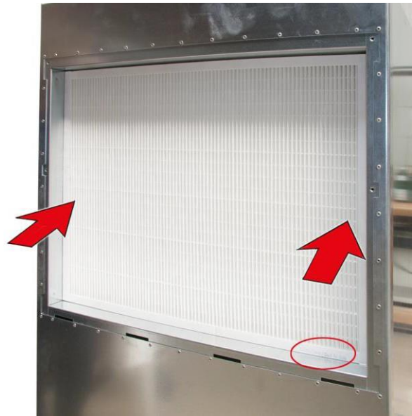
Fig. 12 Inserting the main filter
